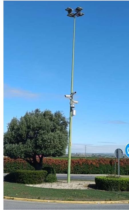
LOCATION 6.1: AFTER THE IMPLEMENTATION
