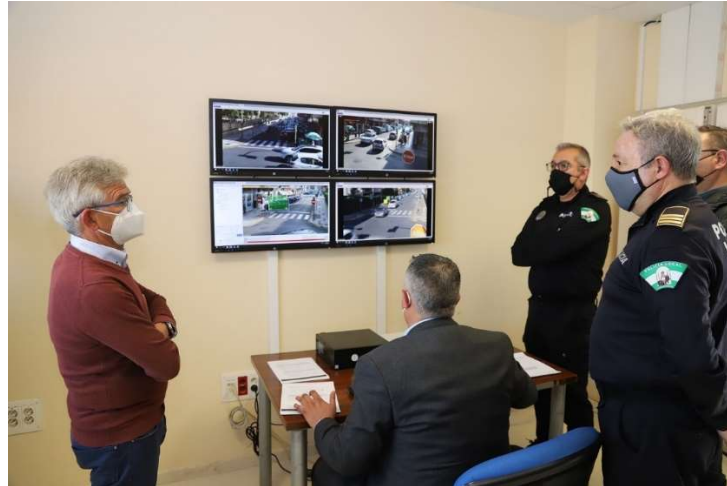
WORKSTATION IN THE POLICE HEADQUARTERS CONTROL ROOM
