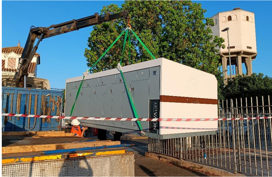
6. INSTALLATION OF THE MODULE NEXT TO THE TOWN HALL
